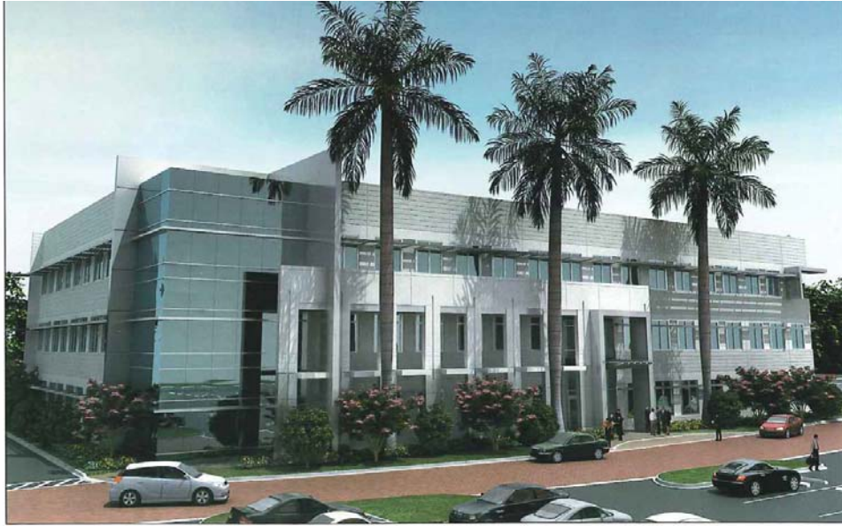
Two future Lynn Financial Center buildings have been pre-certified gold by the U.S. Green Building Council.
