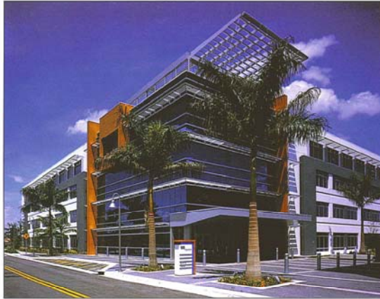
Phase II of 1800 Boca Center is being designed to meet LEED standards.
